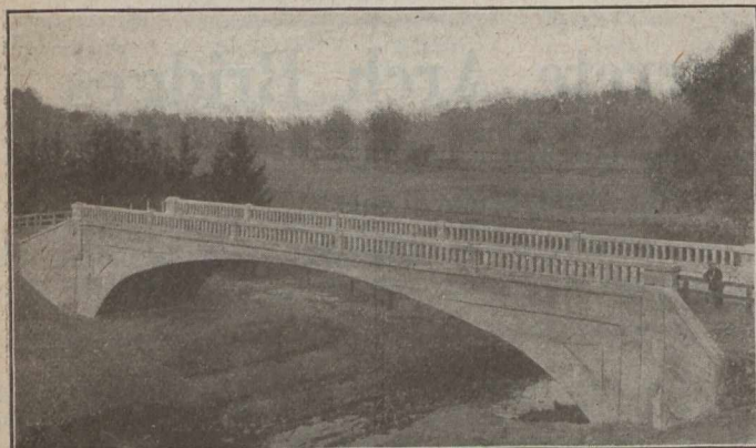
LYNHURST BRIDGE, ST. THOMAS, ONT. (Earth-Filled Arch)
