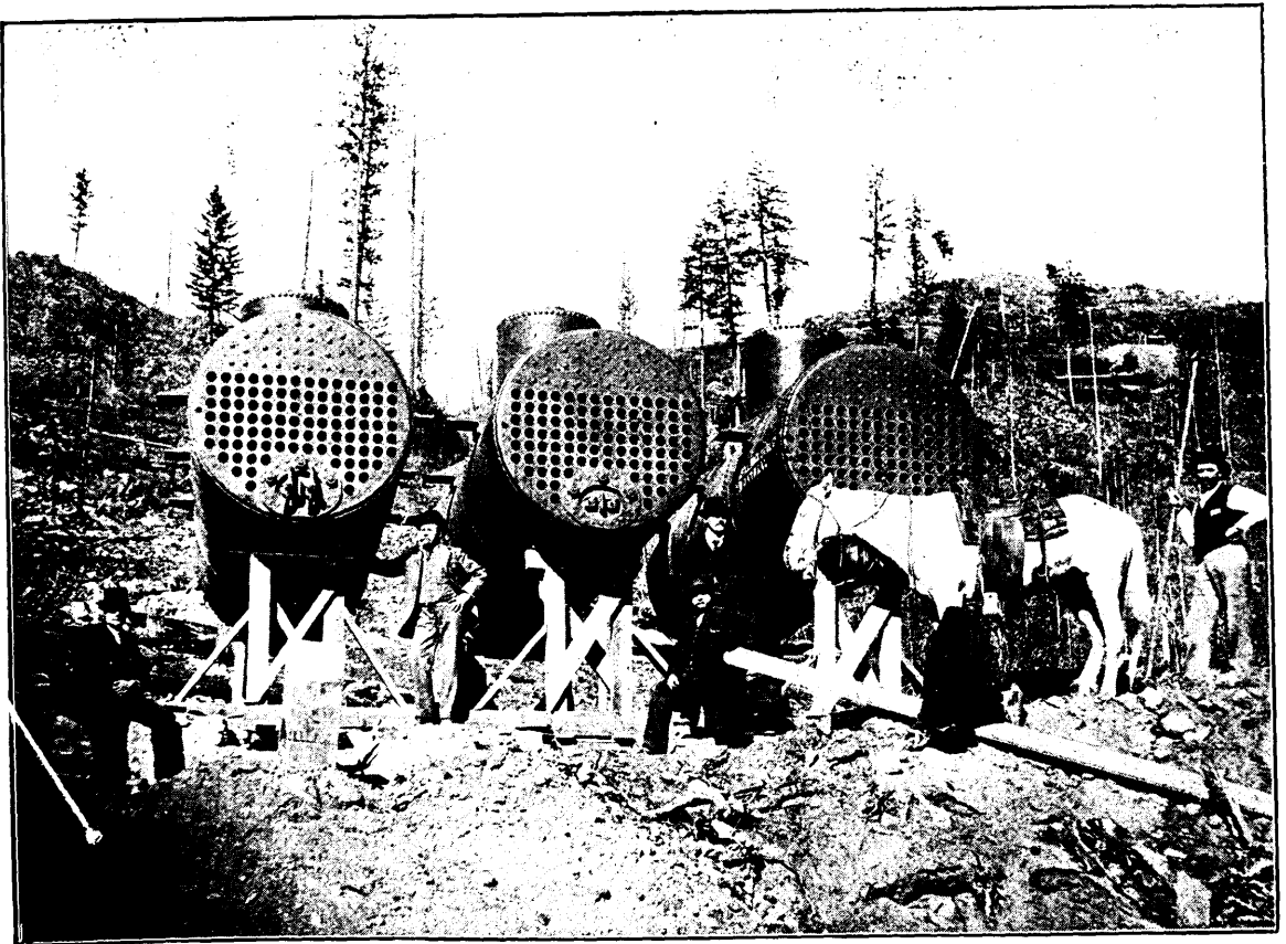
LE ROI NEW COMPRESSOR PLANT, ROSSLAND. (In course of erection.)
