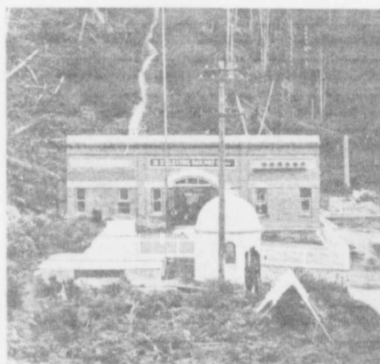
Goldstream Hydro-Electric Plant
