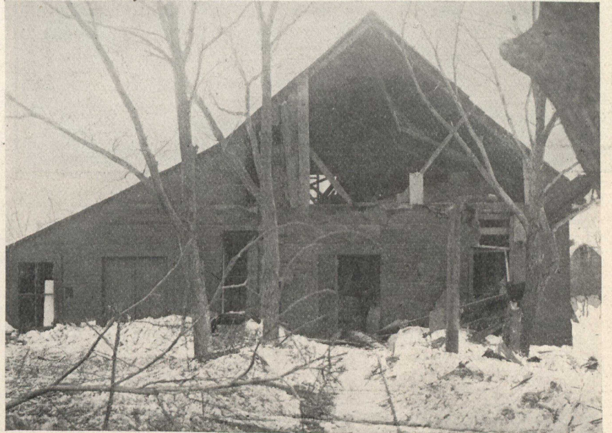
Storage Shed—400 feet distant from the mills that were blown up—wrecked by flying pieces of machinery.
