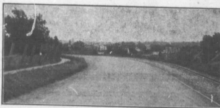
This is Merriton Road in St. Catharines, an important thoroughfare through the manufacturing district between St. Catharines and Merriton, resurfaced with "Tarvia-X," and with "Tarvia-B" and out to 217.
