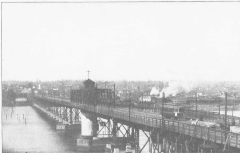
High level steel bridge, Granville Street.
