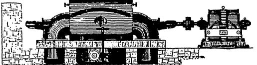
THE accompanying on shows the direct connection of two 20° CROCKER TURINES under 50 ft. head to ELECTRICAL GENERATOR at power station of North Shore Power Co., at St. Narcisse, Que.
