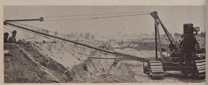
Austin Backfiller at Work on Sewer Trenches.
