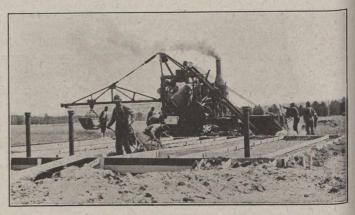
Steam-driven Concrete Mixer, with Boom and Bucket, Working on Latrines.
