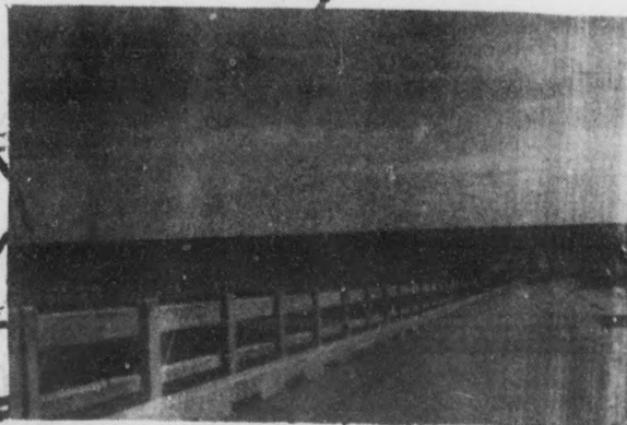
Key West Bridges.
