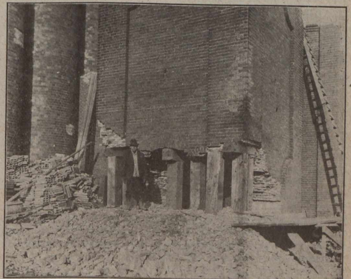
BASE OF CHIMNEY CUT AWAY—TIMBERS READY FOR DYNAMITE CHARGES
