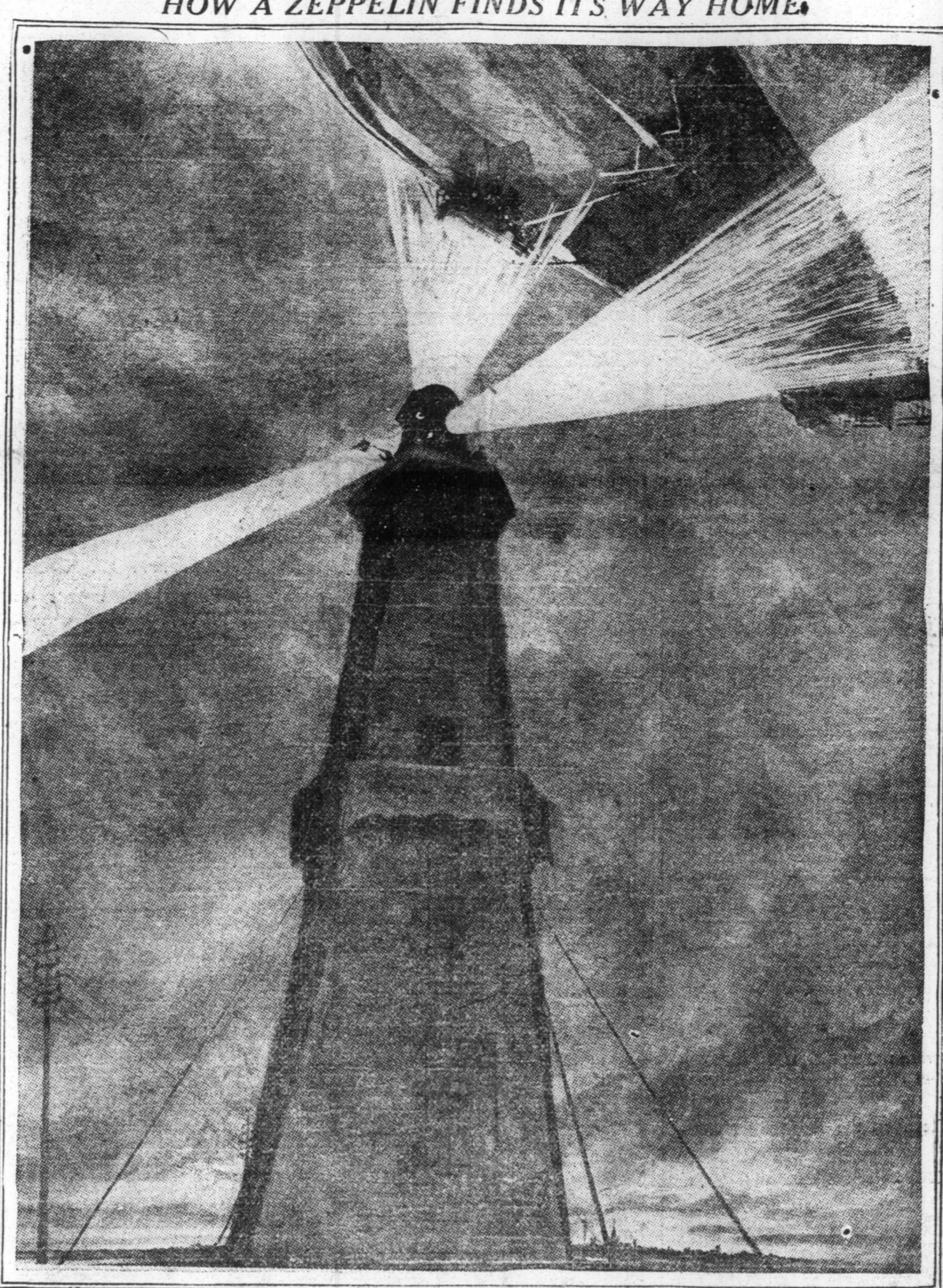
LIGHTHOUSES FOR ZEPPELINS TO GUIDE THEM HOME Toward the end of 1913 the German government promoted a series of trials of new lighthouses to be built for the guidance of aviators flying at night. Many electrical concerns competed, and apparently satisfactory results were obtained. These lighthouses have been erected all over Germany. Some of them project a strong beam of light straight up into the air others show a disappearing light, signaling a number of the flying ground (1-2); for instance, stands for Johannistal, near Berlin; still others, again, are fitted with a rotating light. The above picture, drawn especially for this newspaper, the New York Herald and the London Sphere, shows one of these lighthouses with the keepers signalling to the crew of a passing airship.
