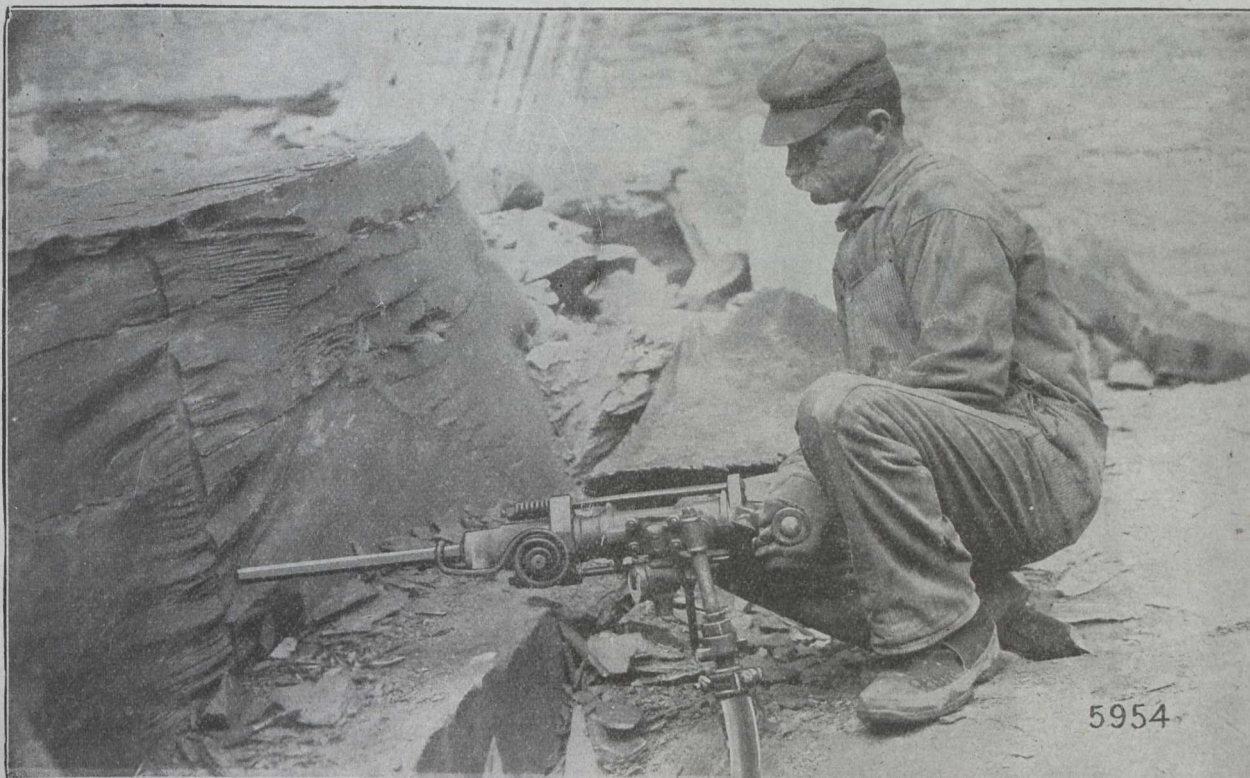
B.C. 430 HAMMER DRILL IN OPERATION
