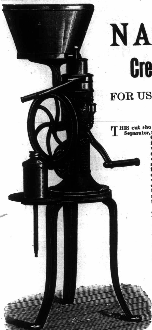
"NATIONAL" NO. 1 HAND POWER. Capacity, 350 to 350 lbs. per hour.
