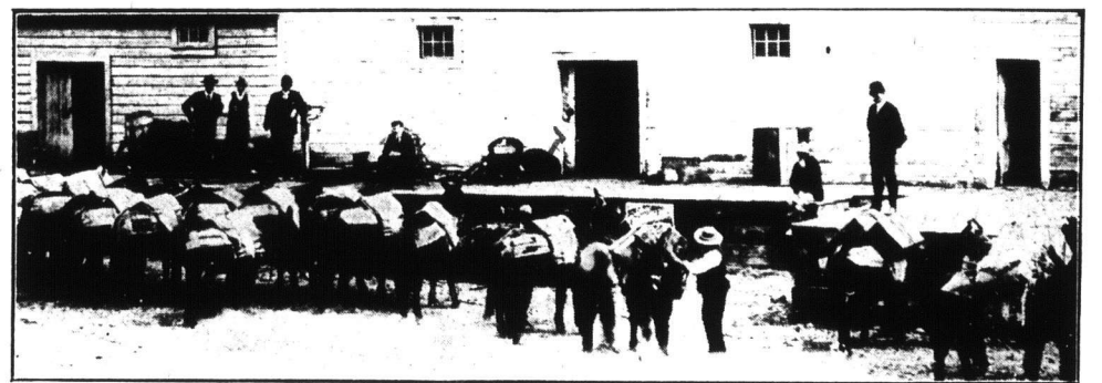
Pack train loaded ready to leave for Northern Interior over Cariboo Road.
