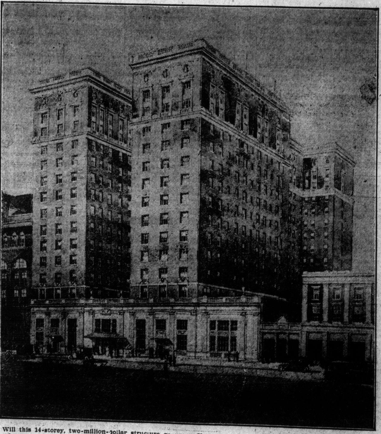
Will this 14-storey, two-million-dollar structure go up on Yonge street in the site of the old Arcade? Or will it not? This question is likely to be settled this morning at the special sitting of the city council, which is to consider the application of the York Hotel Company, represented by W. S. Binnick of the Standard Reliance Mortgage Corporation, for a fixed assessment. The board of control has recommended it. The city treasurer and the assessment commission have approved it. The capital is ready. The action of the council will decide the matter.
