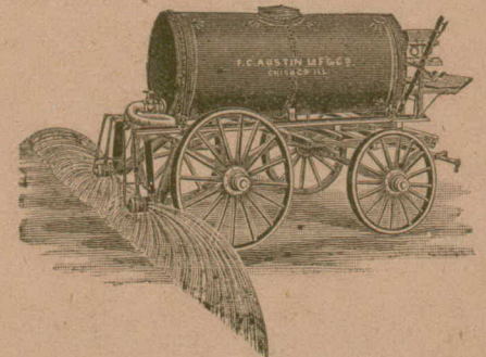
AUSTIN STEEL STREET SPRINKLER
