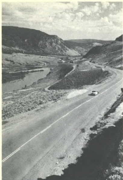
Trans-Canada Highway near Ashcroft, British Columbia
