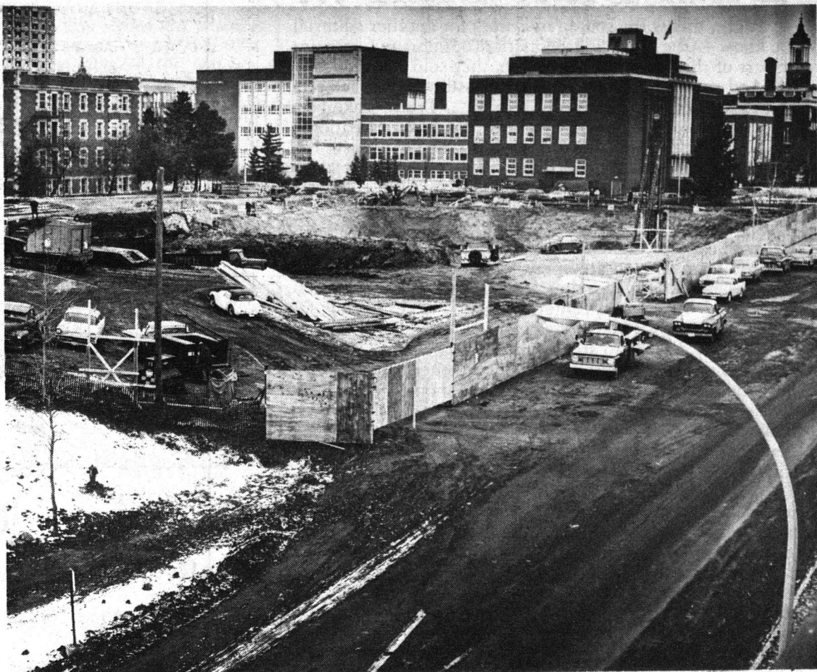
The former site of the Students' Union Building. Construction is proceeding on Gainers' new rendering plant on the site.
