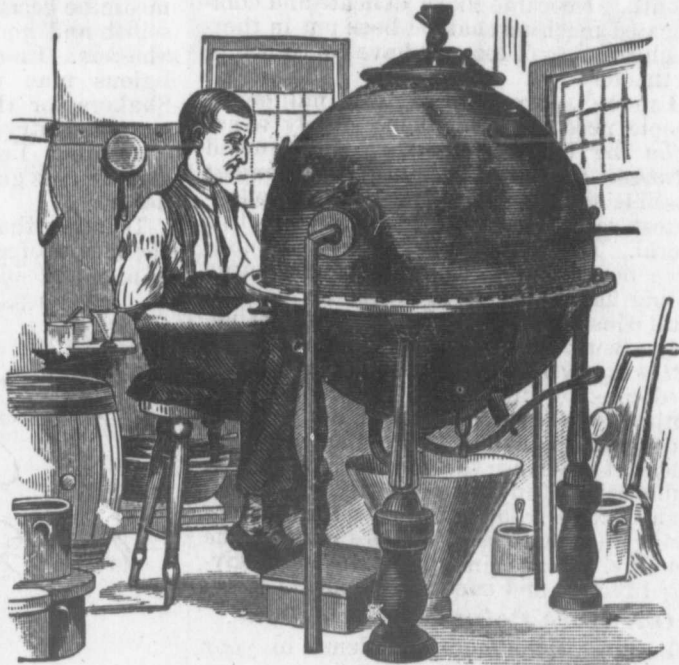
ALONZO HOLLISTER, THE FAMOUS SHAKER CHEMIST, CONCENTRATING MOTHER SEIGEL'S SYRUP, OR SHAKER EXTRACT OF ROOTS, IN VACUUM PAN, MOUNT LEBANON, N. Y.
