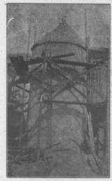
Indispensable on the Small Place. the silo erected by W. L. Smith on his second Durham Co., Ont., as photographed by farm and Dairy shortly after completing monolithic concrete construction, with a st
