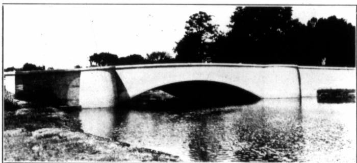
Fig. 27—Auburn Street Bridge, Medford, Mass.
