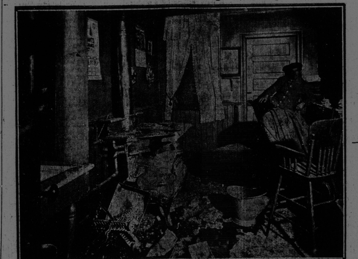
This shows the wreck of a Toronto kitchen, when the householder attempted to light a fire in the range during the cold snap. There was a complete blow up—the water pipes were frozen in the front of the stove and they caused the burst. Albert Plenty was nearly killed.
