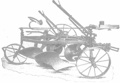
Our new SCOTCH CLIPPER HIGH-LIFT GANG has foot-lift and release, also hand-release for use when walking. These features have been perfected on our plow, and a small boy can operate easily, whether
