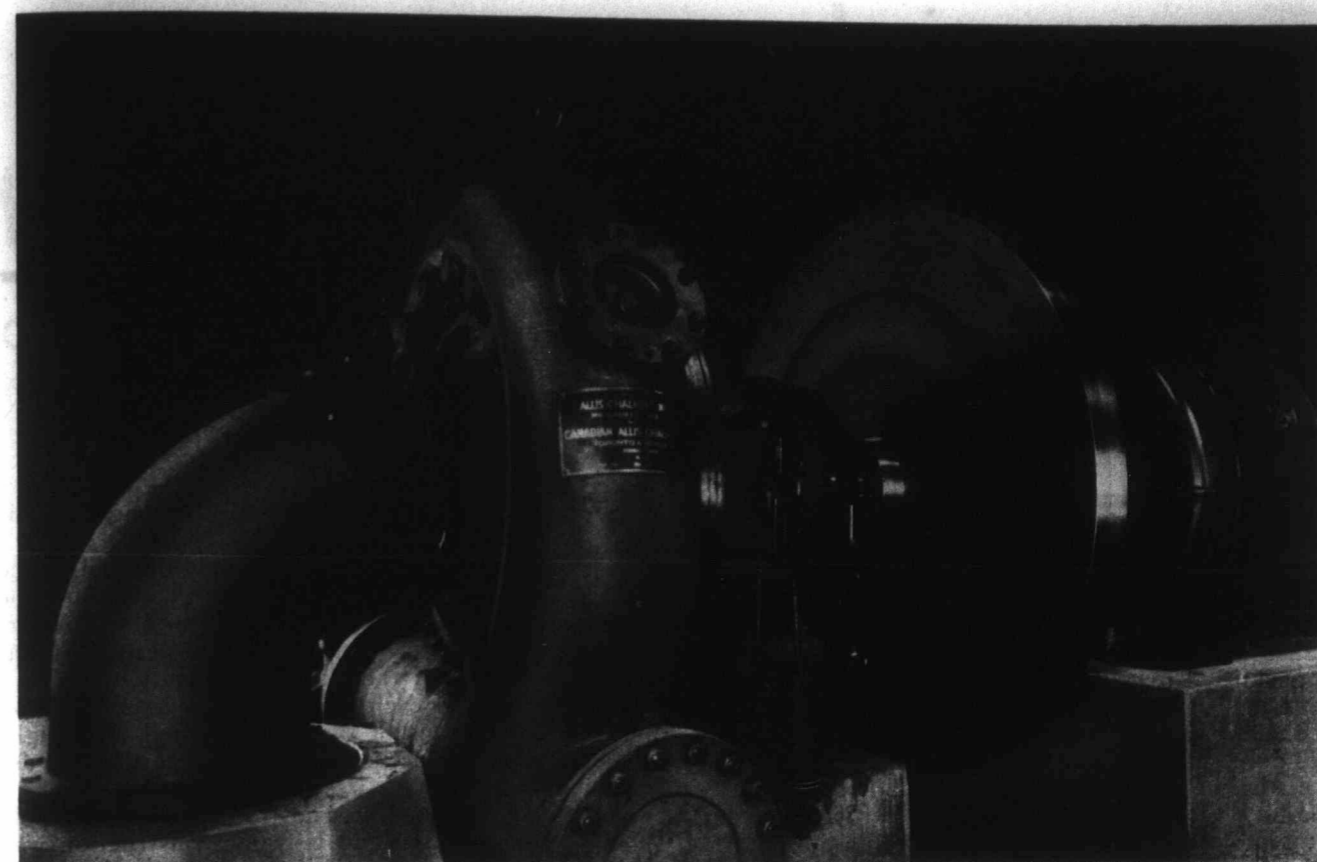
Above: The new 1,000 hp. hydro-electric unit in the Pioneer Mine takes up little space.
