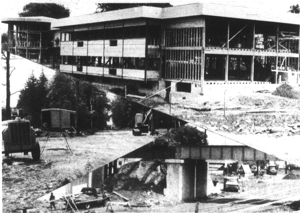
Time Waits For No Man — That fact is evident as the Mississauga area receives a major face-lifting job. Above is seen the new Port Credit Legion, the Mississauga Rd., near the intersection of Indian Rd., and No. 10 highway, both of which are undergoing reconstruction.
