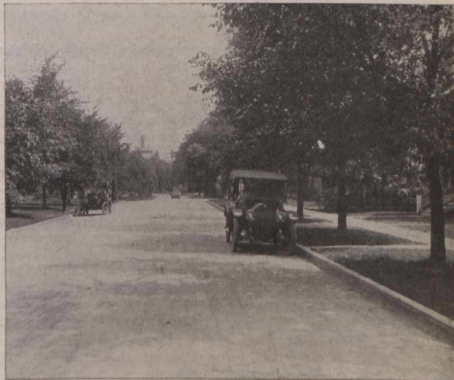
Finished Dolarway Pavement.
