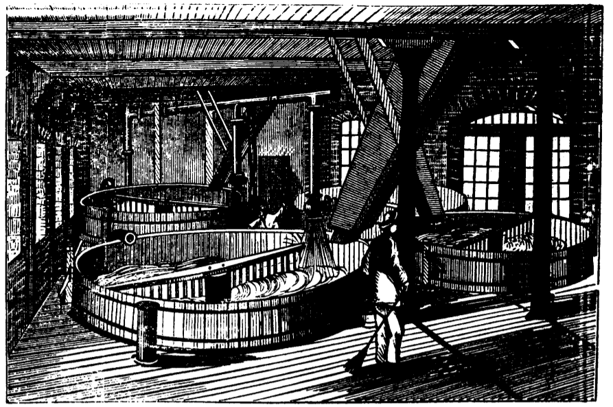
No. 6.—MASHING ROOM.
