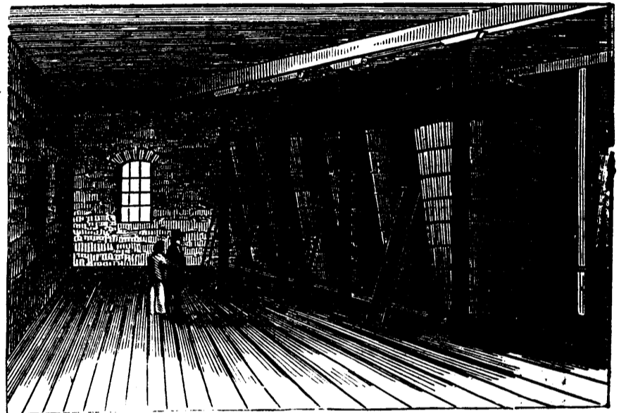
No. 9.—RECTIFYING ROOM ; ONE SECTION.
