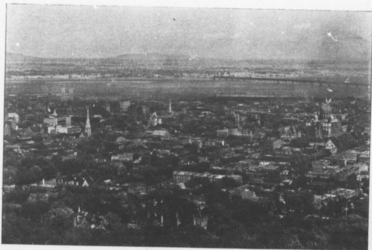
PARTIAL VIEW OF MONTREAL OF TO-DAY.
