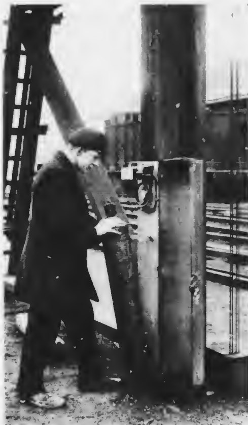
PUTTING IN A FILLED ACCUMULATOR (OLD TYPE OF BOX).
