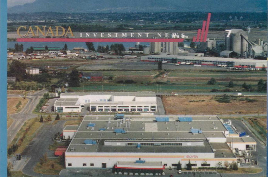
Set in a 25-acre site, the 19,000 square-metre plant at Delta, British Columbia, supplies Toyota facilities in Canada, the United States and Japan.
