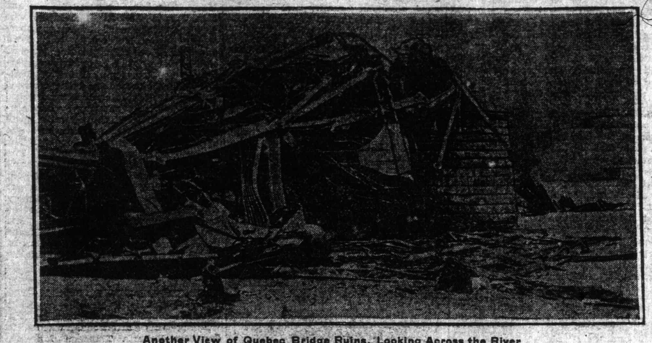
Another View of Quebec Bridge Ruins, Looking Across the River
