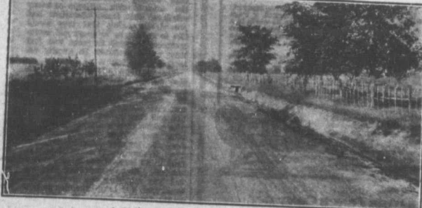
A Clay Road that is Kept Good by Dragging.
