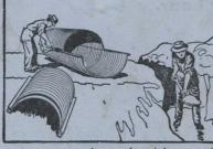
are made from Toncan metal which is 99.94% pure iron and which has double the life of any other known metal for the purpose.
