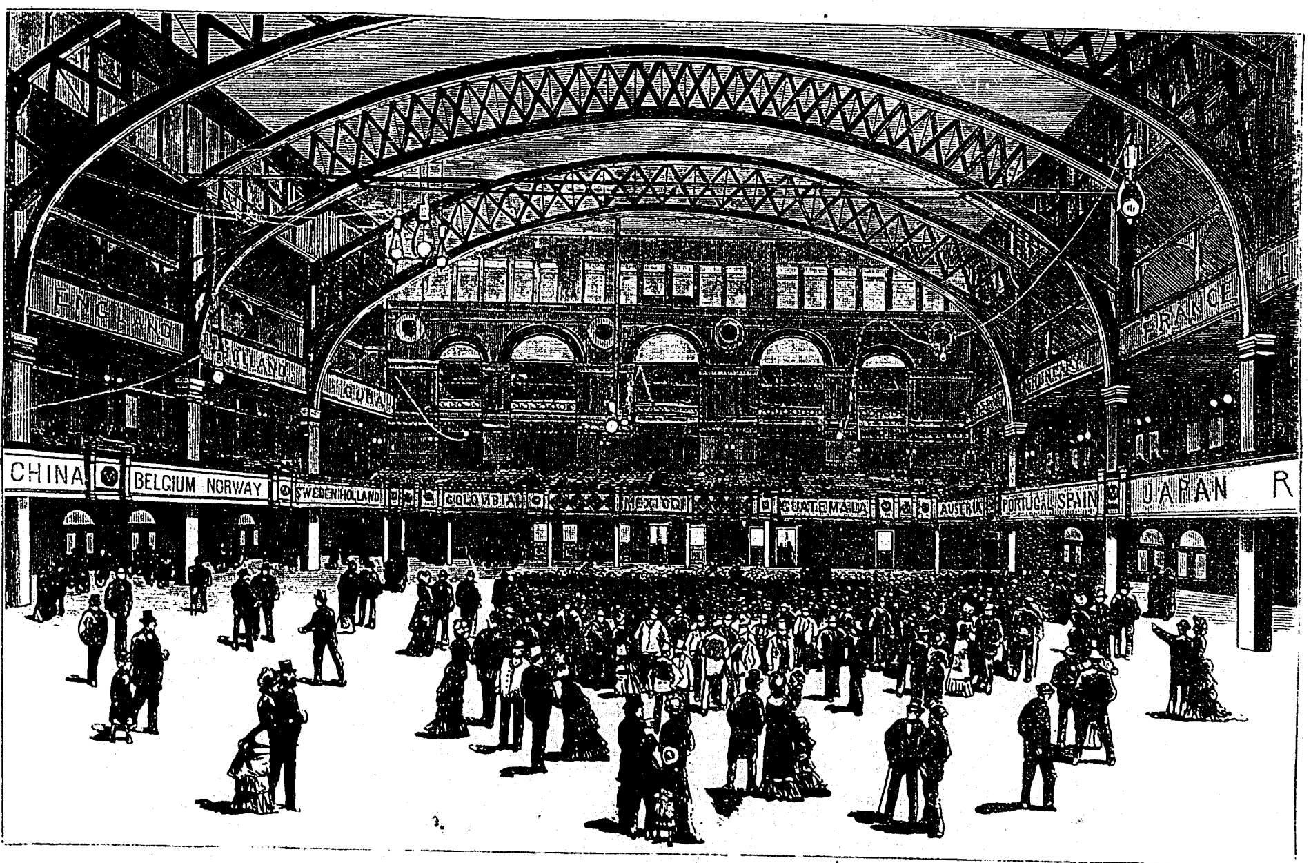
INTERIOR OF THE EXPOSITION BUILDING. THE GREAT FOREIGN EXHIBITION AT BOSTON.
