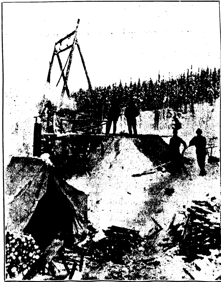
WINTER WORK ON BONANZA CREEK, YUKON.
