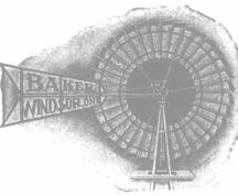
The wheel is built on a hub revolved on a long stationary steel spindle. As a result there is less friction.
