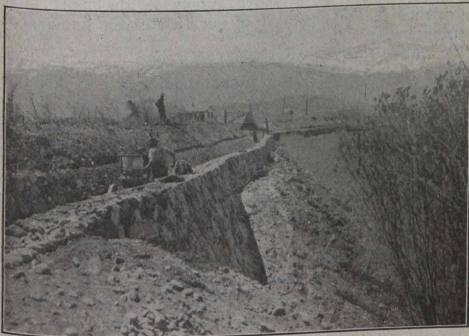
Fig. 1.—Showing Retaining Wall on Downhill Side of Canal
