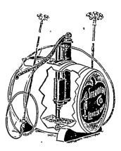
**THE SPRAMOTOR** is a machine designed for the application of all kinds of spray mixtures and paints, being operated by Engine, Horse or Man Power. The illustrations show the Hand Power Machine that was awarded First Place in the Canadian Government Contest, and the Gasoline Power Outfit as operated by the Dominion Government Fruit Division this year, to demonstrate to the growers the best way to raise a profitable crop of Fruit.
