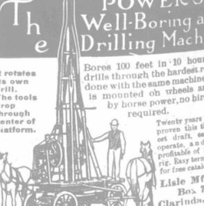
Bores 100 feet in 10 hours, and drills through the hardest rock, all done with the same machine, which is mounted on wheels and run by horse power, no hired help required.
