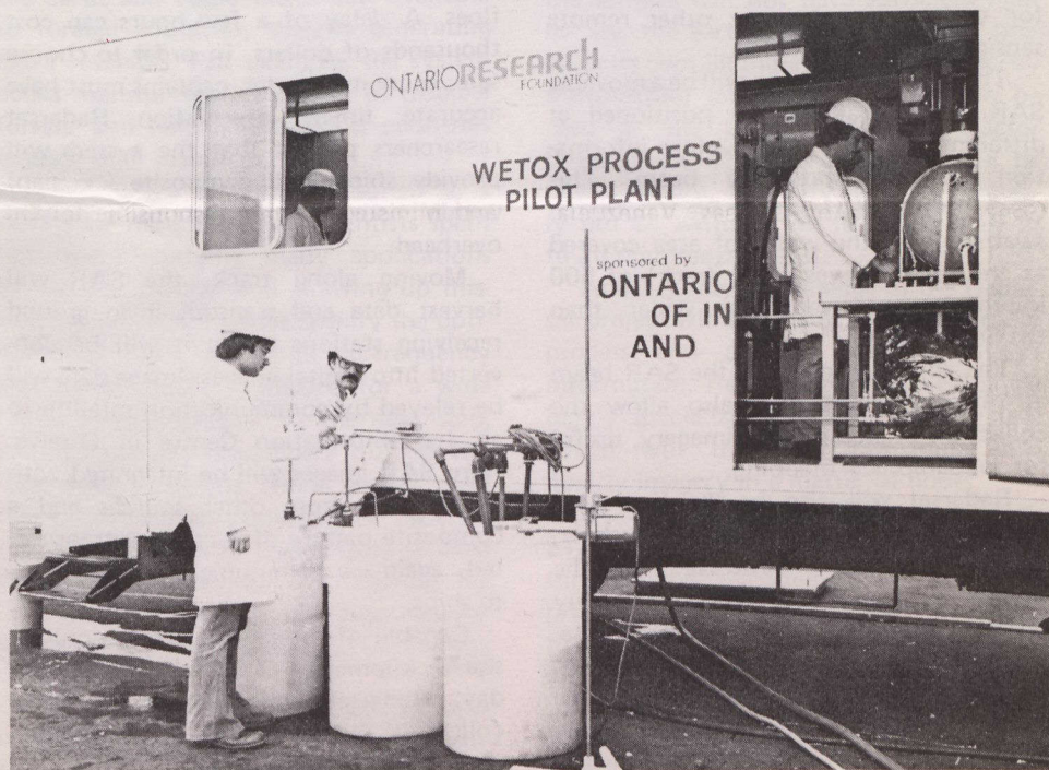
Pilot plant: Ontario Research Foundation's 2 273 litre mobile unit demonstrates capabilities of the Wetox system, a breakthrough in the disposal of toxic organic waste.
