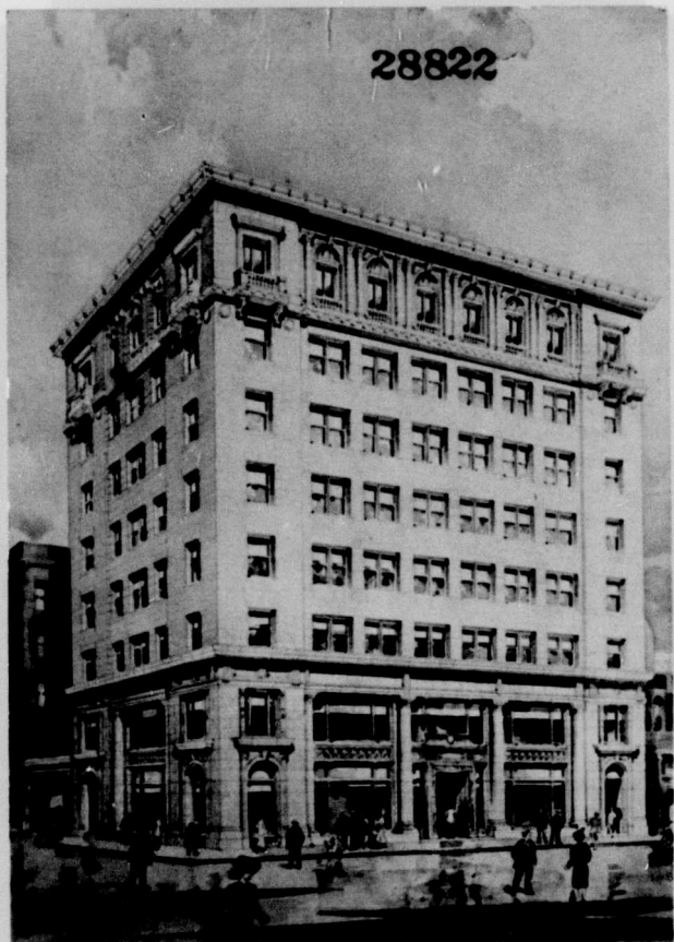
"SALADA" TEA CO.'S New Building in course of construction, corner of Berkeley and Stuart Streets, Boston, Mass. When completed, it will be the finest Tea Warehouse in the world.
