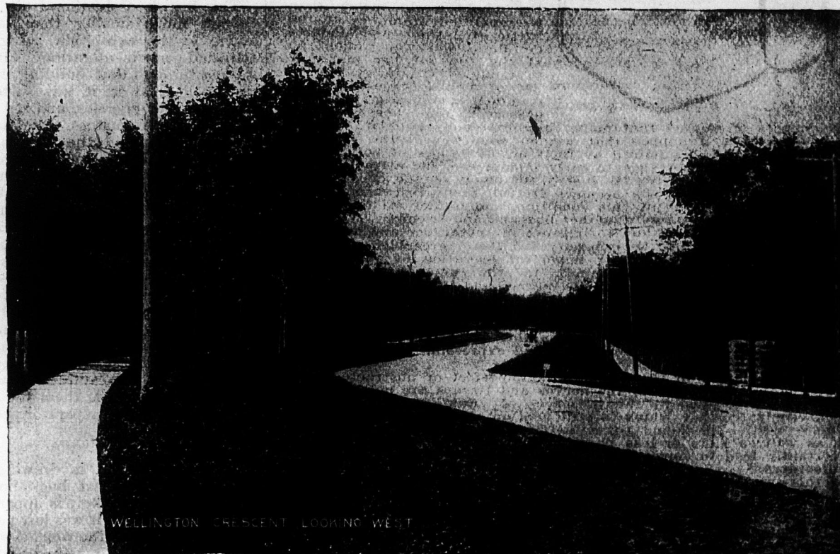
Wellington Crescent Driveway, Looking West.
