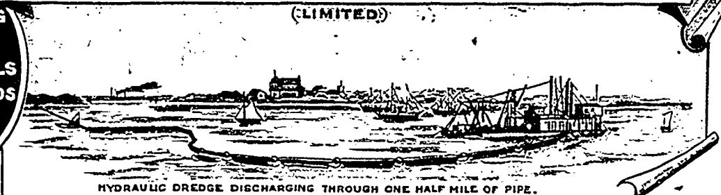
HYDRAULIC DREDGE DISCHARGING THROUGH ONE HALF MILE OF PIPE.
