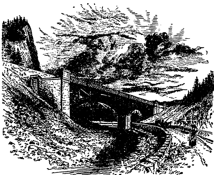
ASHWOOD DALE BRIDGE, NEAR BUXTON.
