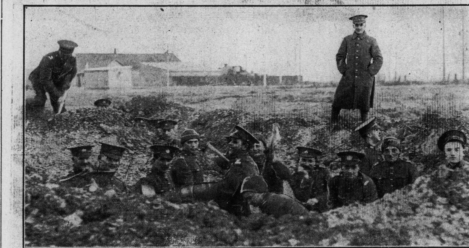
SOLDIERS DIGGING DEEP IN OLD MOTHER EARTH. Happy and contented these men seem, though hard at work gaining experience in the digging of trenches. Won't you volunteer to-day and help them?
