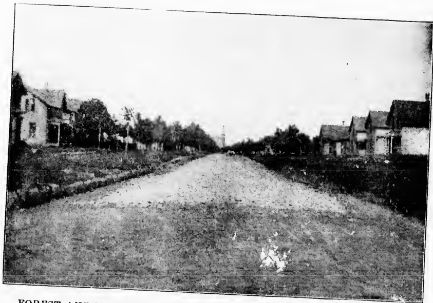
FOREST AVENUE, ST. THOMAS. --The above photo shows the street in process of construction, May, 1896.
