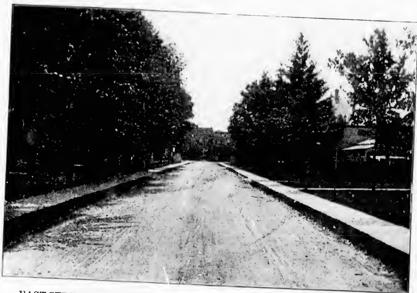
EAST STREET, ST. THOMAS. --The roadway is twenty-two feet wide, curbed with 3x10 cedar and made of crushed stone ten inches in depth at the centre and seven at the curb after consolidation with a heavy road roller. The sidewalks are four feet wide, of pine. The street was improved in 1895, and the above photograph taken May, 1896.
