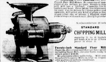
Acso manufacture 20 inch STANDARD CHOPPING MILL capacity 15 to 35 bushels per hour, 6 to 10 or 12 horse power to drive it.
