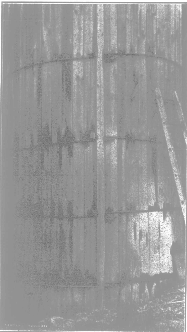
A Good Way of Fastening Hoops on a Stave Silo.
