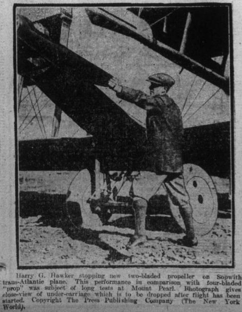
Harry G. Hawker stepping new two-bladed propeller on Sopwith trans-Atlantic plane. This performance in comparison with four-bladed "prop" was subject of long tests at Mount Pearl. Photograph gives close-up view of under-carriage which is to be dropped after flight has been started. Copyright The Press Publishing Company (The New York World).
