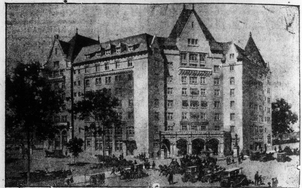
The new Grand Trunk Pacific Hotel, "The Macdonald," Edmonton, will be a notable addition to the Dominion list of palatial hotels.
